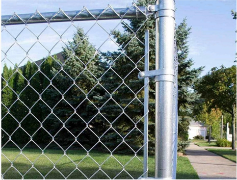
Tension Bar Assembly
